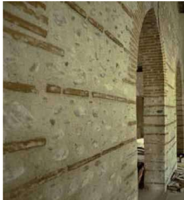
Historic internal wall repaired with Natural Hydraulic Lime mortar
