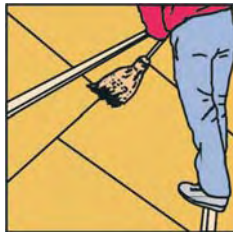
Clean surface with a brush. Surface must be dry to ensure adhesion.
