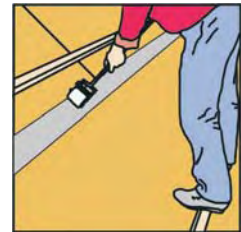
Press tape on firmly using a seam roller.
